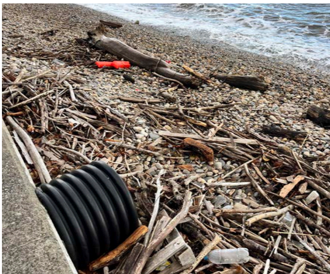
↓ Debris at the Cornfield Point Sea Wall - Old Saybrook
