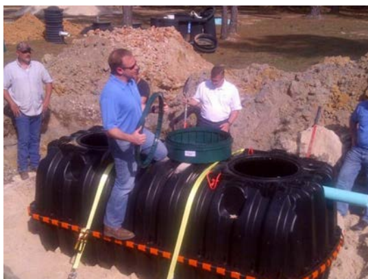
↑ Securing a plastic septic tank with straps
