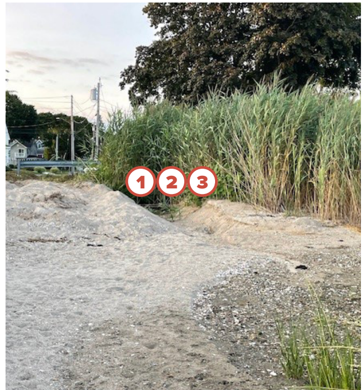
⬆ Existing condition of the outfall at Old Sea Lane.
