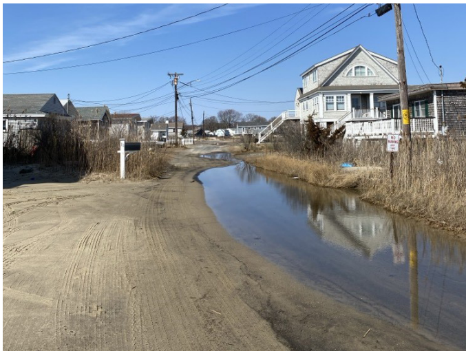
↓ Barnes Rd Flooding - Old Saybrook
