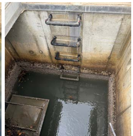
↑ Inside of the Chalker Beach Tide Gate
