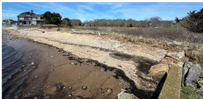
↑ Erosion at west return of the 43 Pettipaug Avenue seawall. Hightide breach allows ocean access to Old Fenwick inland wetland.
