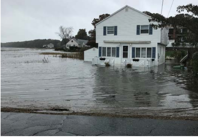
Great Hammock Rd Flooding - Old Saybrook
