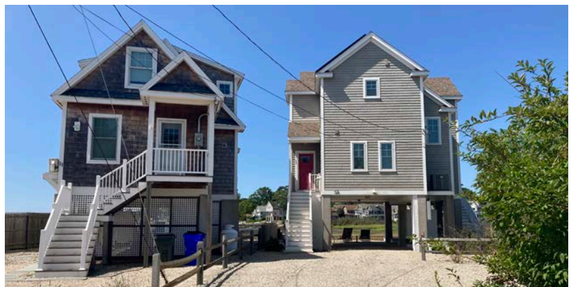
↑ Elevated structures on Beach Road W, Old Saybrook
