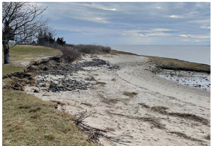
↓ Shoreline Town Beach Erosion - Clinton
