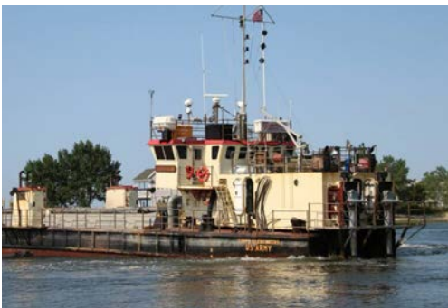
↑ Dredging of Patchogue River, Westbrook, 2022
