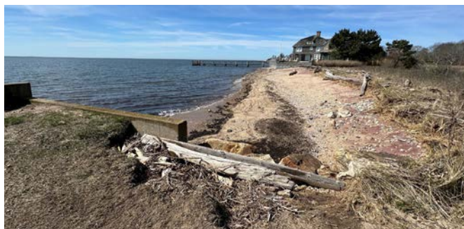
↑ Erosion at west return of the 43 Pettipaug Avenue seawall. Hightide breach allows ocean access to Old Fenwick inland wetland.
